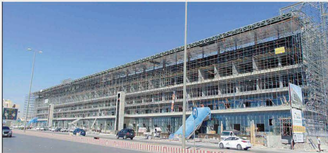
Raden Center - Olaya Road - Riyadh
