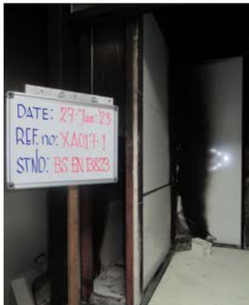
After Fire Test
