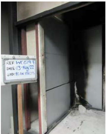
After Fire Test
