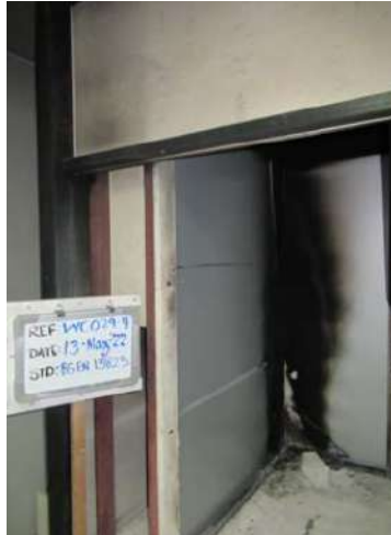
After Fire Test
