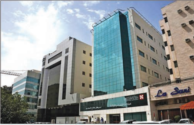
Administration Building - Riyadh
