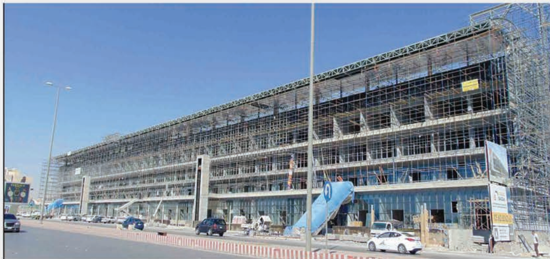
Raden Center - Olaya Road - Riyadh
