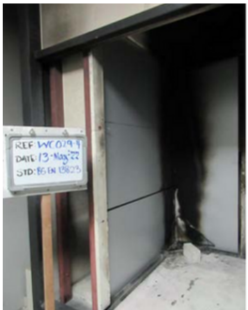
After Fire Test
