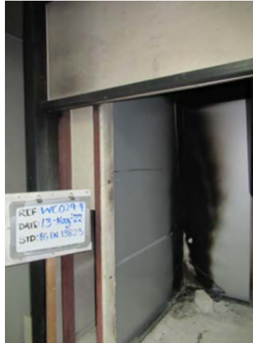
After Fire Test
