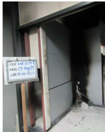
After Fire Test
